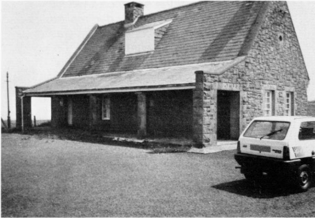
Front of Crosslaw guardhouse before conversion. From owner's archive
